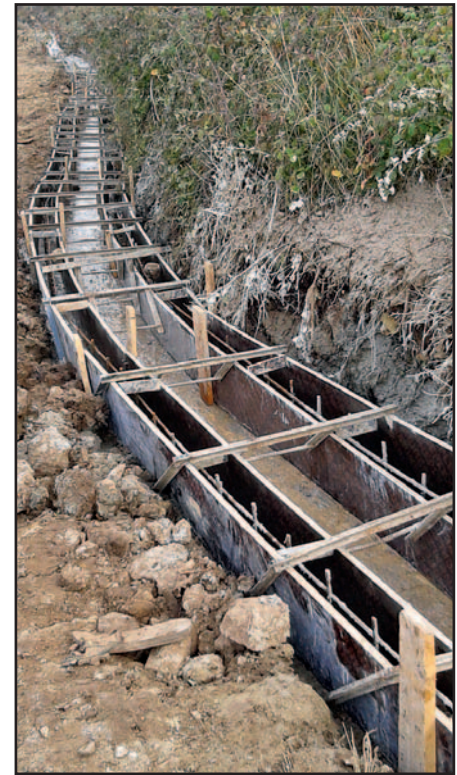
Irrigation Channel Akkar - Adelnord
