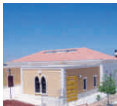
Yater Municipal Building
