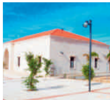
Ansar Municipal Building
