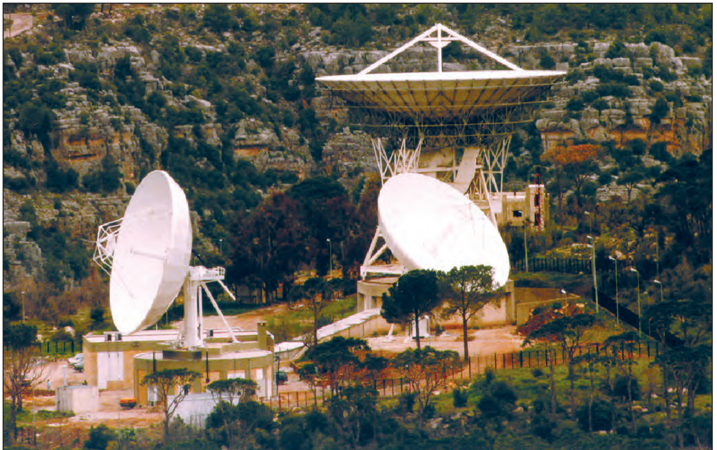
Construction & installation of international telephone exchange: Jourret El Ballout-Metn
