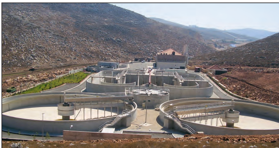
Nabatieh wastewater treatment plant
