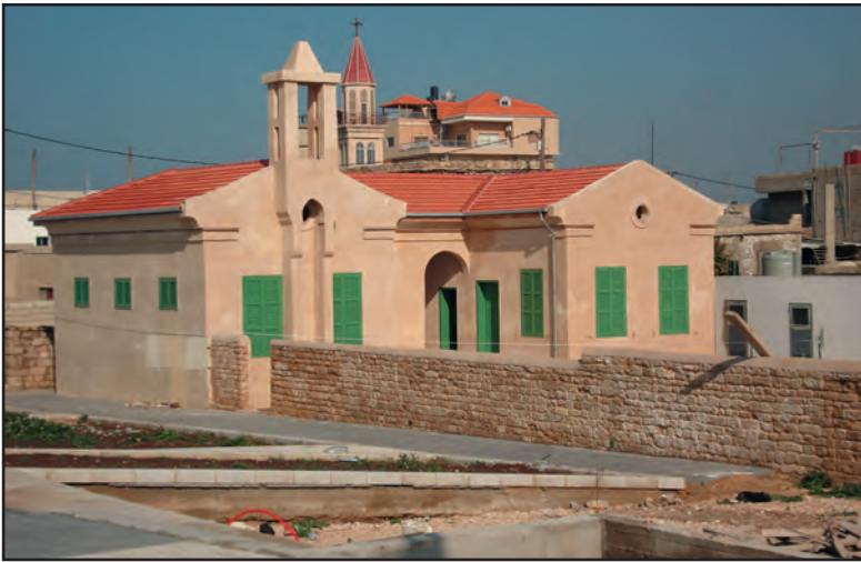
Rehabilitation of Archeological sites in Tyre.
