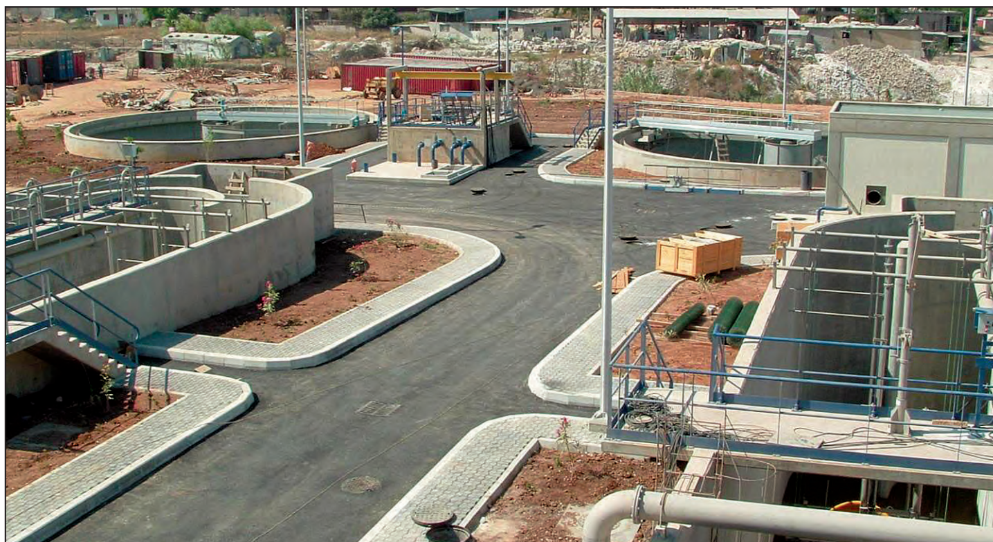
Chekka wastewater treatment plant
