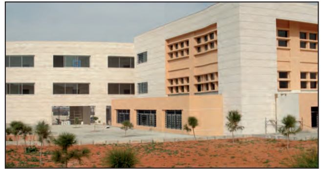
The Technical school (Al Kaa)
