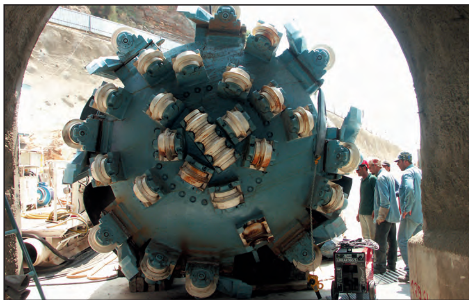
Potable water supply for Kesrwan coastal region.
