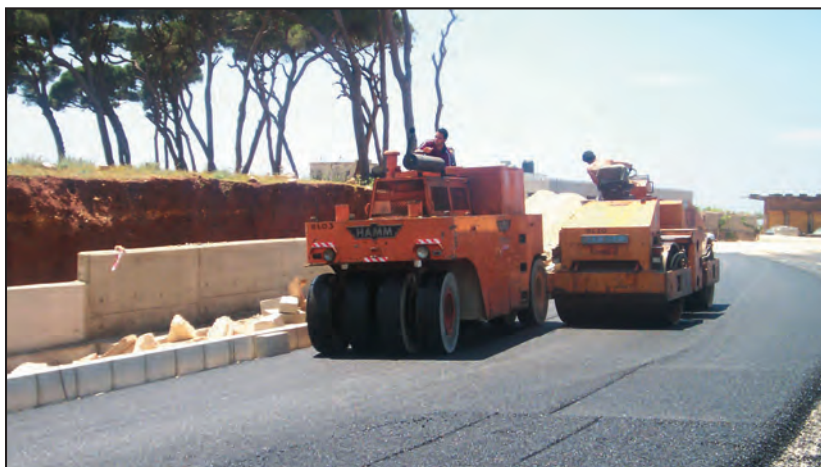
Rehabilitation of Bchamoun, Aramoun Road.
