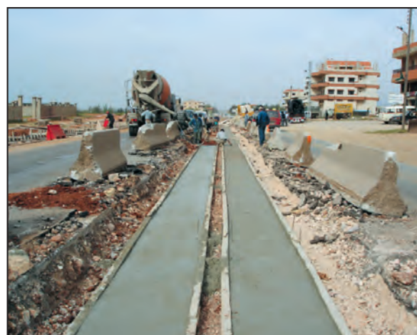
Rehabilitation Chtoura Masnaa Highway.
