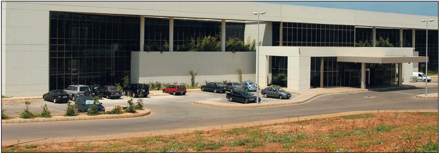
General aviation building
