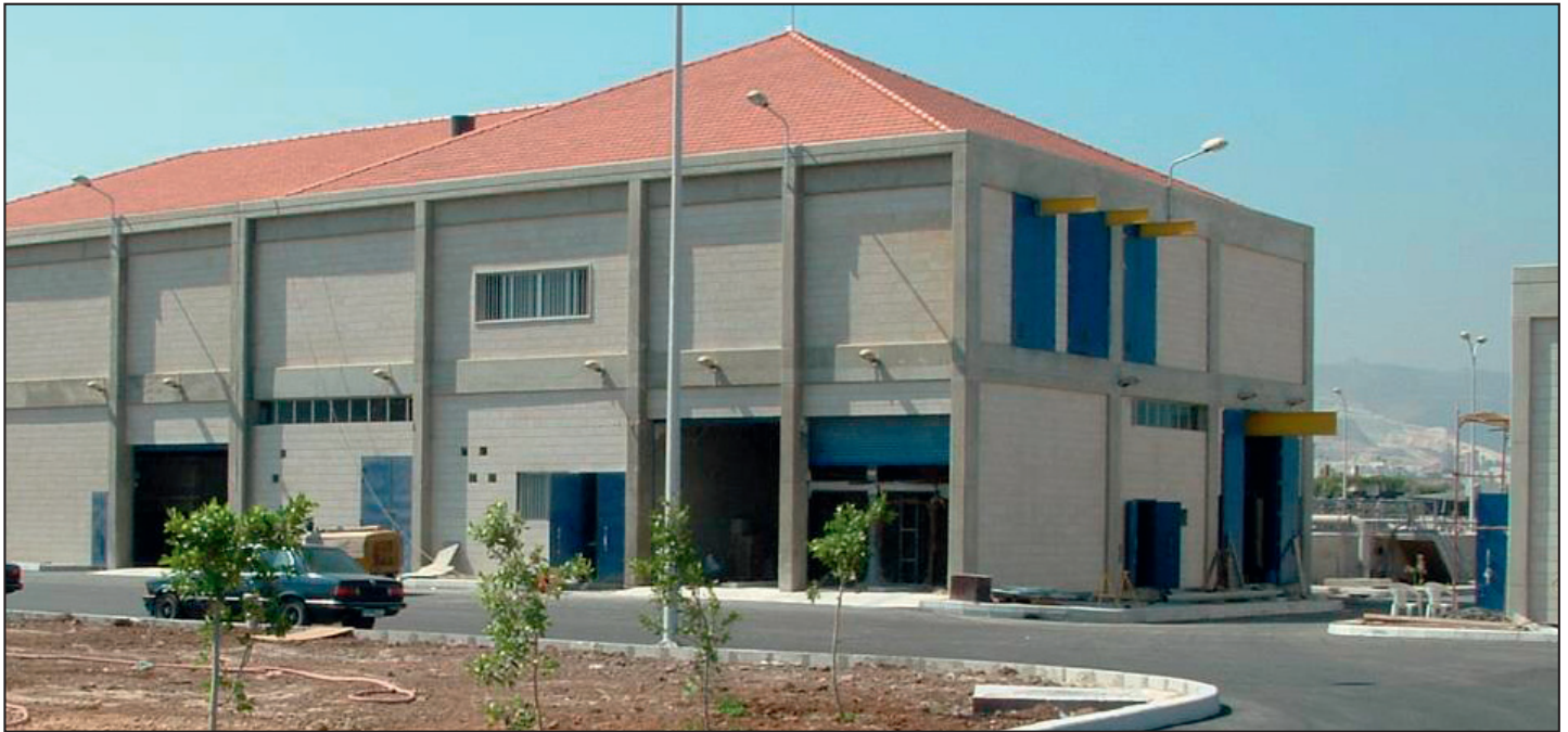
Wastewater treatment plant in Chekka
