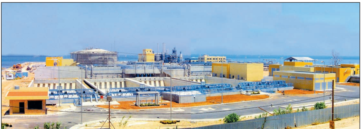
Wastewater treatment plant in Tripoli
