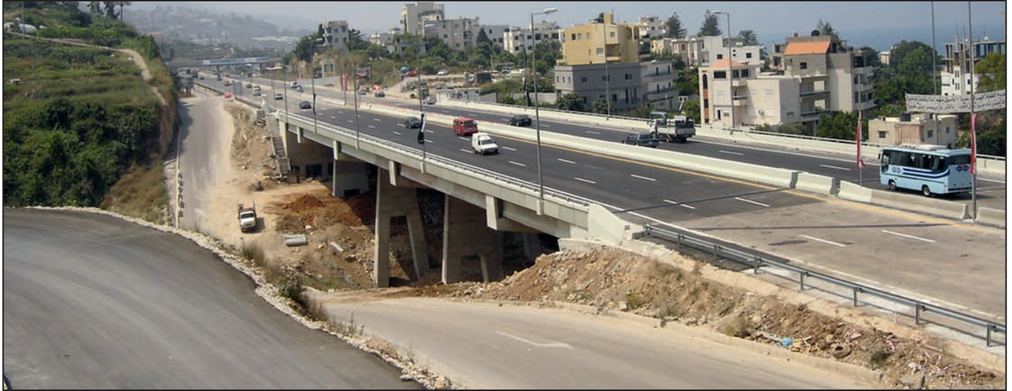
El Fidar Bridge
