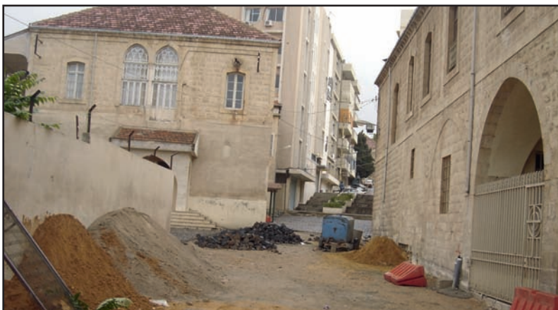
CHUD - Rehabilitation of Historic Building - Baalbeck
