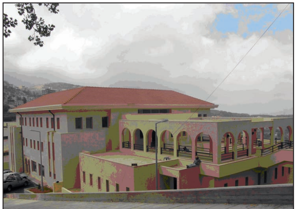
Kaemakamiet Dannieh Building
