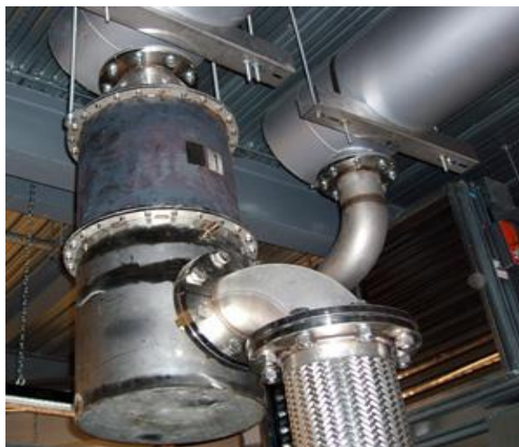
Exhaust systems incorporating diesel particulate filters
