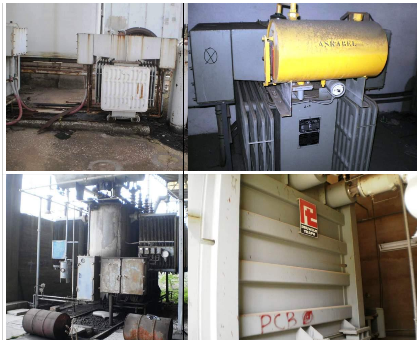
Photograph 5-1: Out-of-service Askarel Transformers and PCB-containing Capacitors in the Zouk Site (Geoflint 2012).
