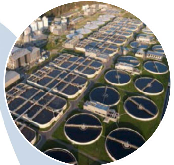
WWTP & Greywater treatment plants
