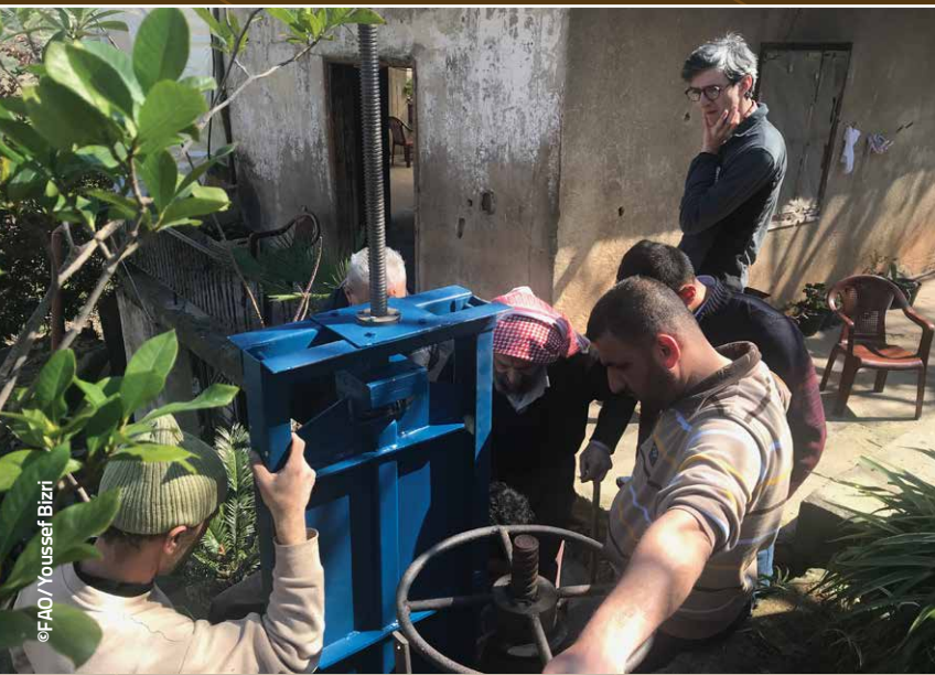
Figure 8: Inception of installed gate with farmers
