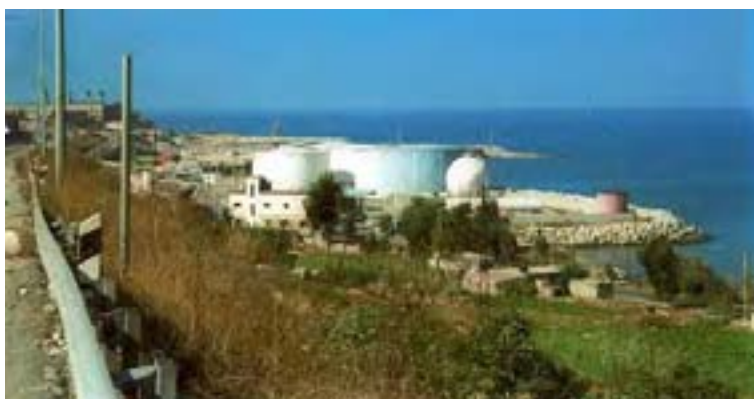
Photo 39: Industry along the coastline; Petroleum bulk terminal and power- generating plant in Jiyeh
