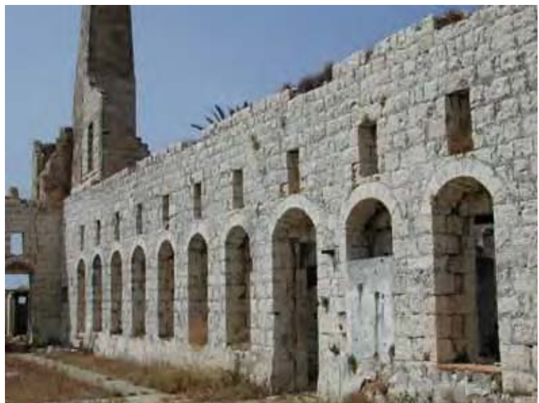
Photo 68: Remains of silk factory at Damour. The building maintains the links with the town's important industrial past
