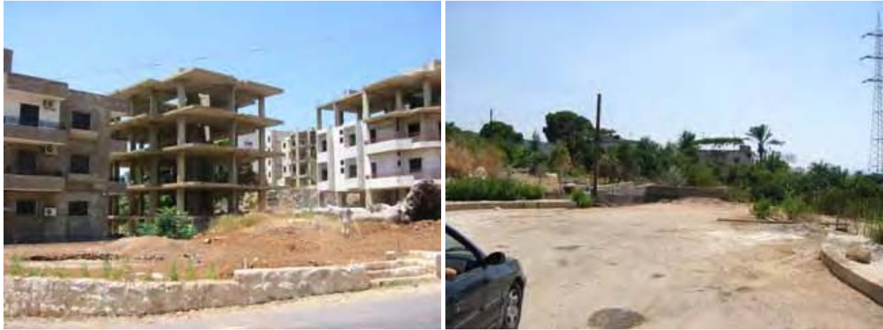
Photo 13, Photo 14: Examples of construction works
