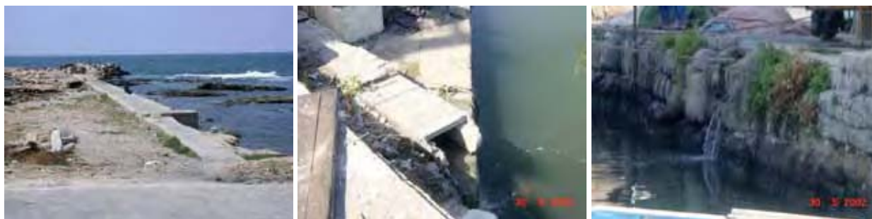
Photo 42, Photo 43, Photo 44: Outfalls and channels discharging wastewater directly into the sea in Sour
