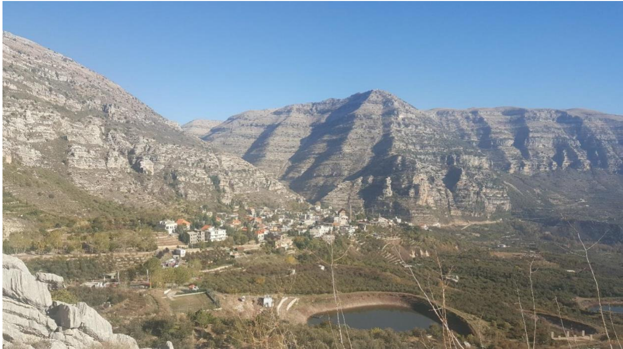
Irrigation pond in Ehmej. (Photo by PMSPL II staff)
