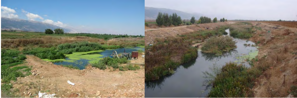
Riverbed dammed for irrigation pumping (Ghazze), Over-widened riverbed but not maintained (Joub Jenine) regardless of water quality
