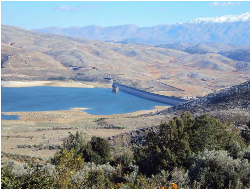
Qaraoun Dam storing flows from the Litani River in the southern Bekaa Valley
