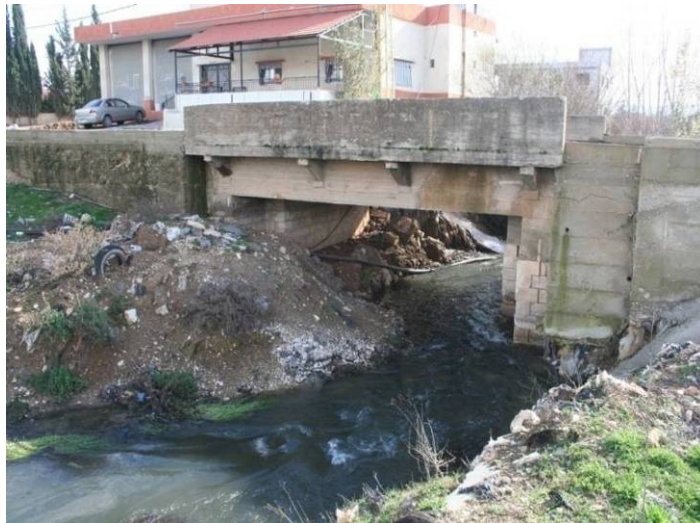
Photograph 7.9: Dumping of Construction Rubble
