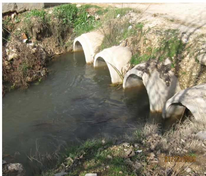
Photograph 7.2: Section of Bridge/Culvert (L2 UP) showing 4 Pipes near Haouch Er Rafqa
