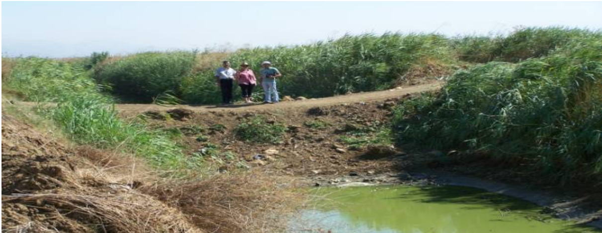
Photograph 7.11: Embankment Weirs for Irrigation
