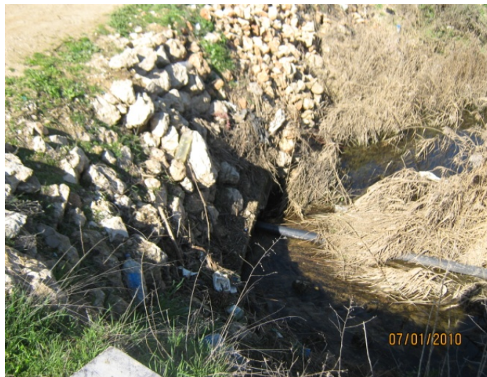
Photograph 7.6: Culvert (F5) on Faregh Tributary
