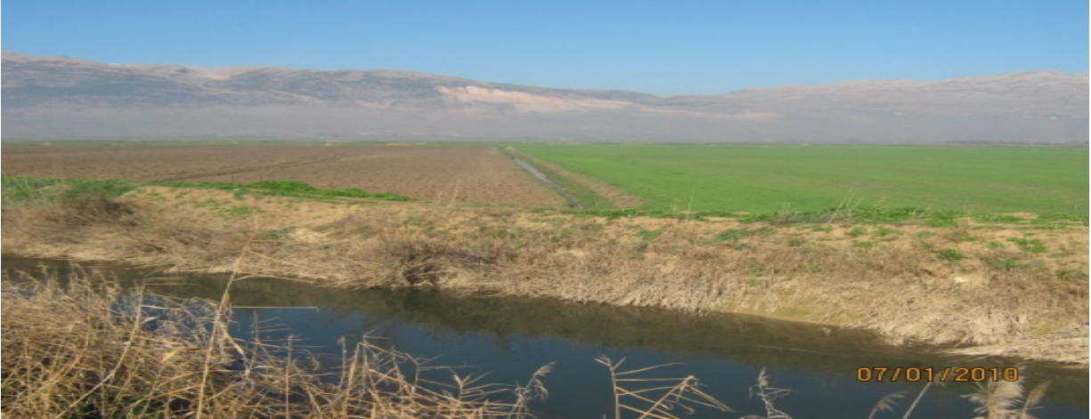
Photograph 7.10: Heightened River Sides via Levees
