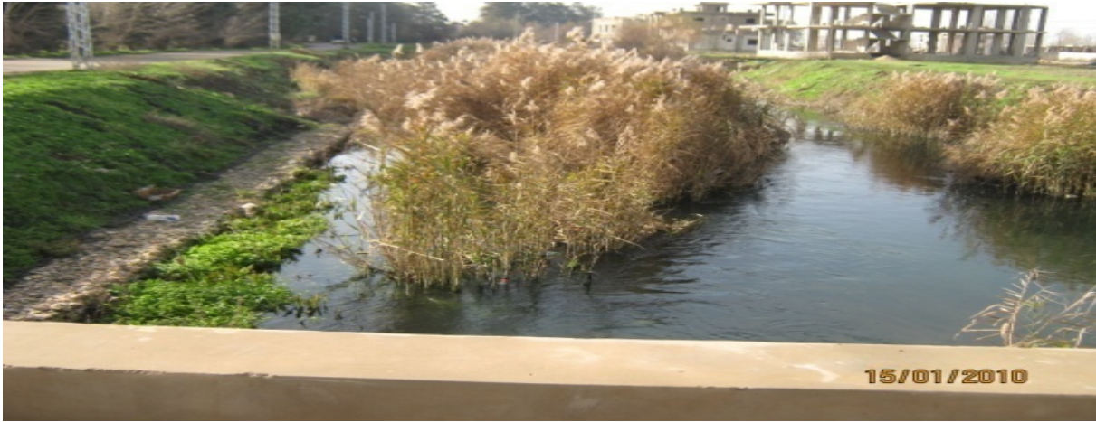
Photograph 7.12: Growing Vegetation in River Bed
