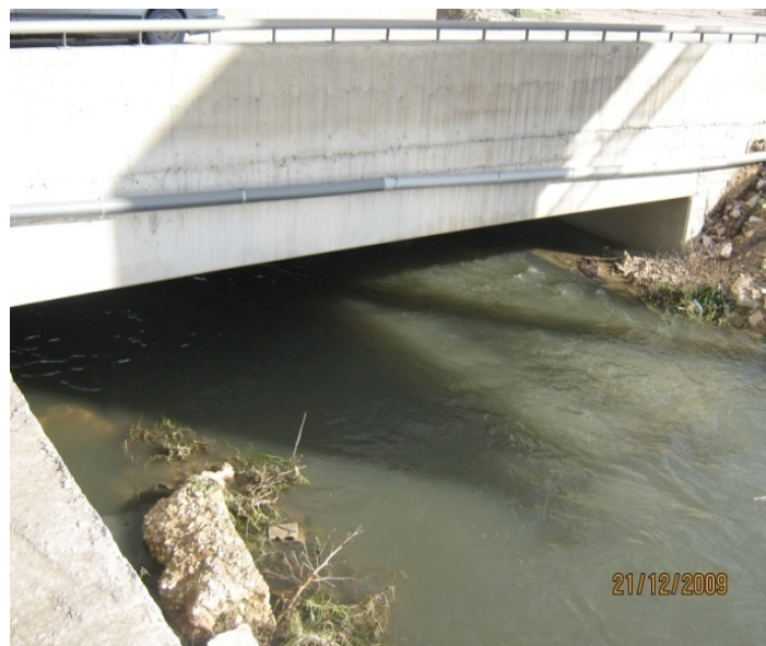
Photograph 7.4: Bridge (L6) on Ablah Road
