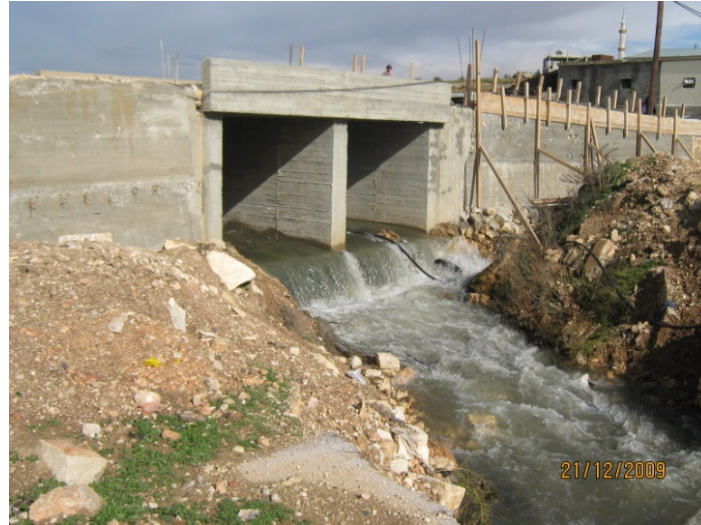
Photograph 7.3: Bridge (L3) on Road that Leads to Bednayel showing Level Difference
