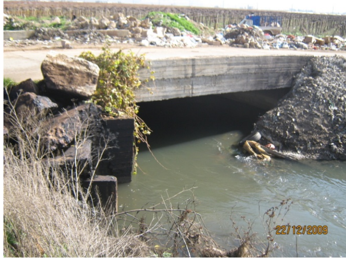
Photograph 7.5: Bridge (L9) in Mkhat El Laouz
