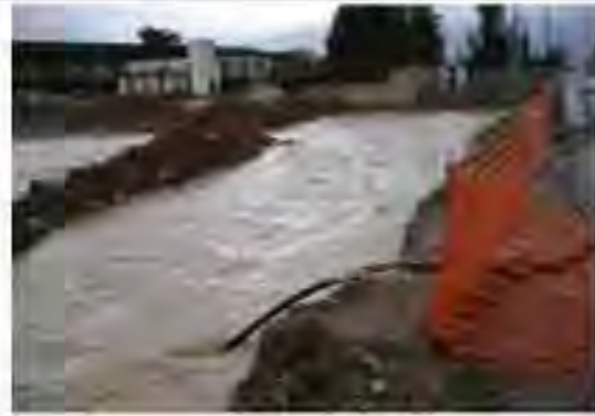
Bridge Downstream during a Seasonal Flood
