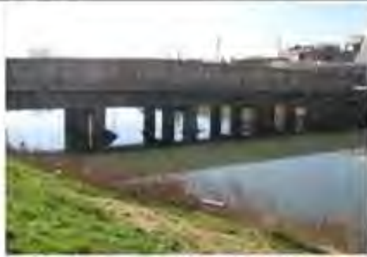
Bridge from Upstream
