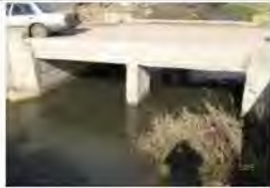
Bridge on Main Road (2 Culverts - Width = 2m)
