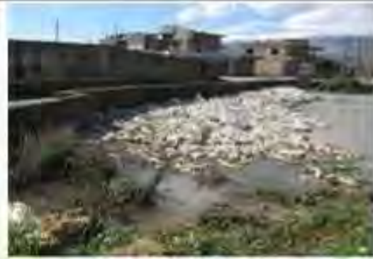
Bridge from upstream after a seasonal flood in 2010
