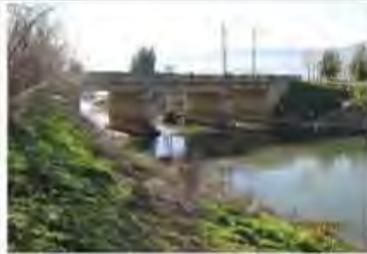
Bridge from Upstream
