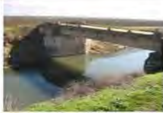
Old Bridge from Upstream
