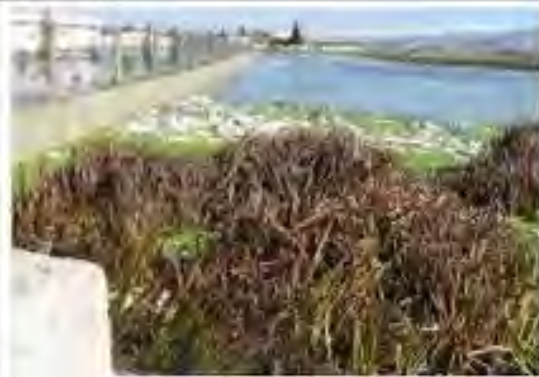
Solid Waste Upstream the Bridge
