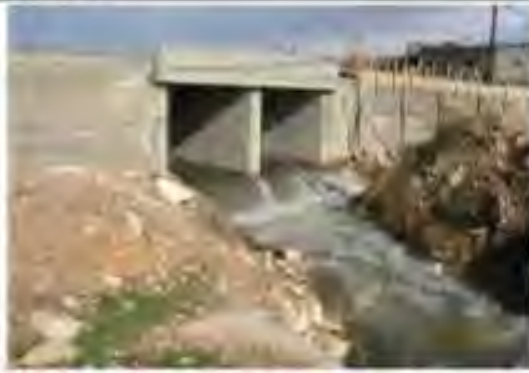
Bridge (Downstream) Wing Walls under construction
