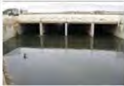
Bridge from Upstream
