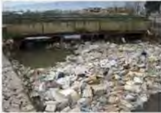
Pipe under bridge blocking Solid Waste
