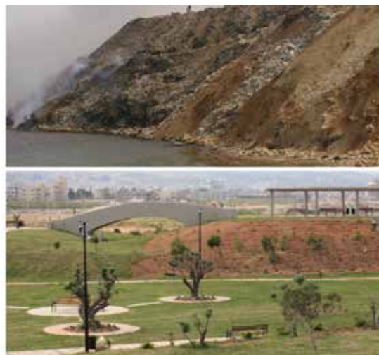
Rehabilitation of the Saida dumpsite into a public park
