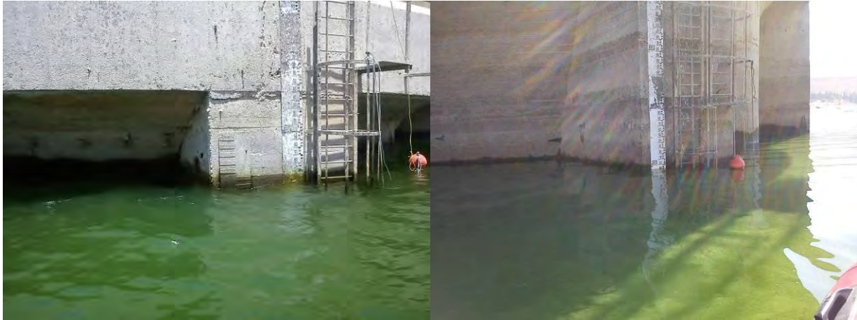
Figure 5 Water Level Scale attached to the spillway
